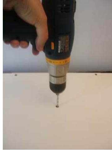
Drill the Holes
